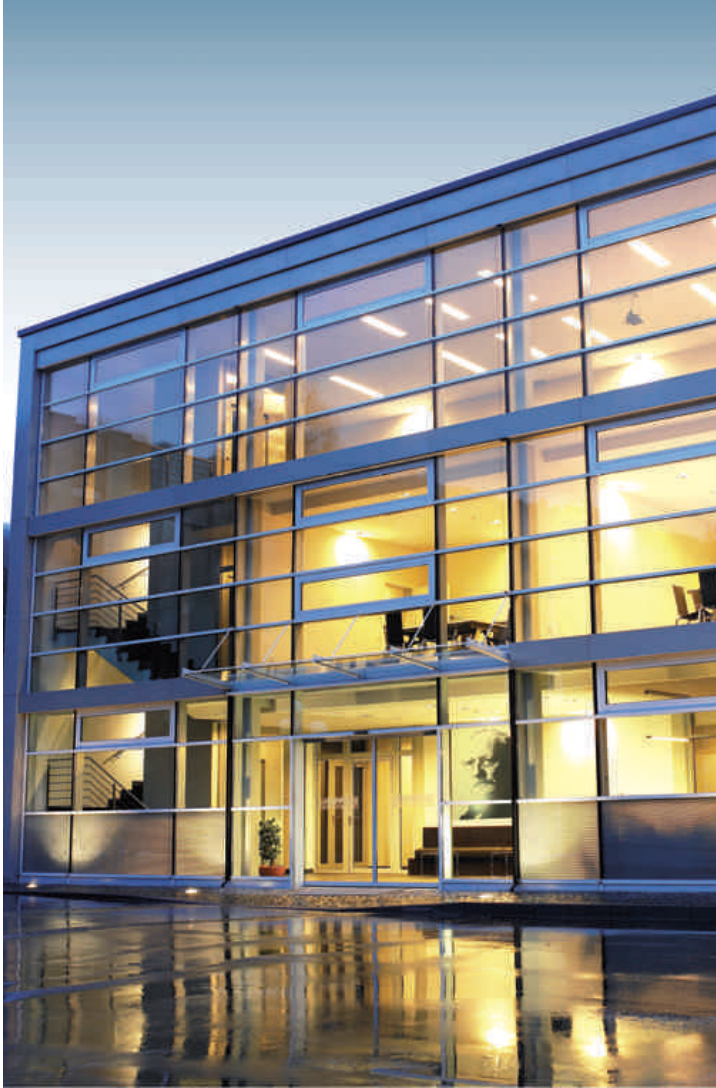
HOPPECKE company headquarters in Brilon, Germany
