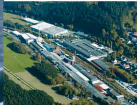
Production plant Brilon-Hoppecke
