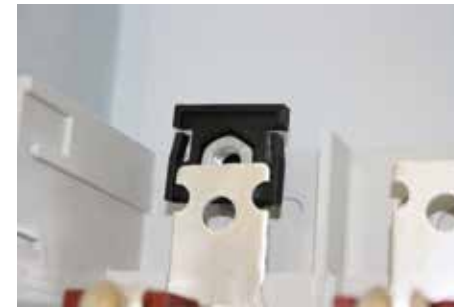
Figure 2: Fixing the nut below the flange connection
